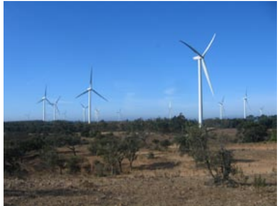
Figure 2 : Wind turbines (2MW) in the study area location
