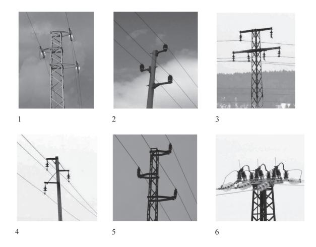
Fig. 2. Surveyed Different 20 kV pole configurations
